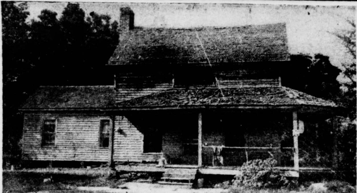
The old Hutchison house is of sturdy log construction underneath the weatherboarding. The ell to the left has been added in comparatively recent years. The story and half section has been standing well over a century. (Herald Staff Photo).
