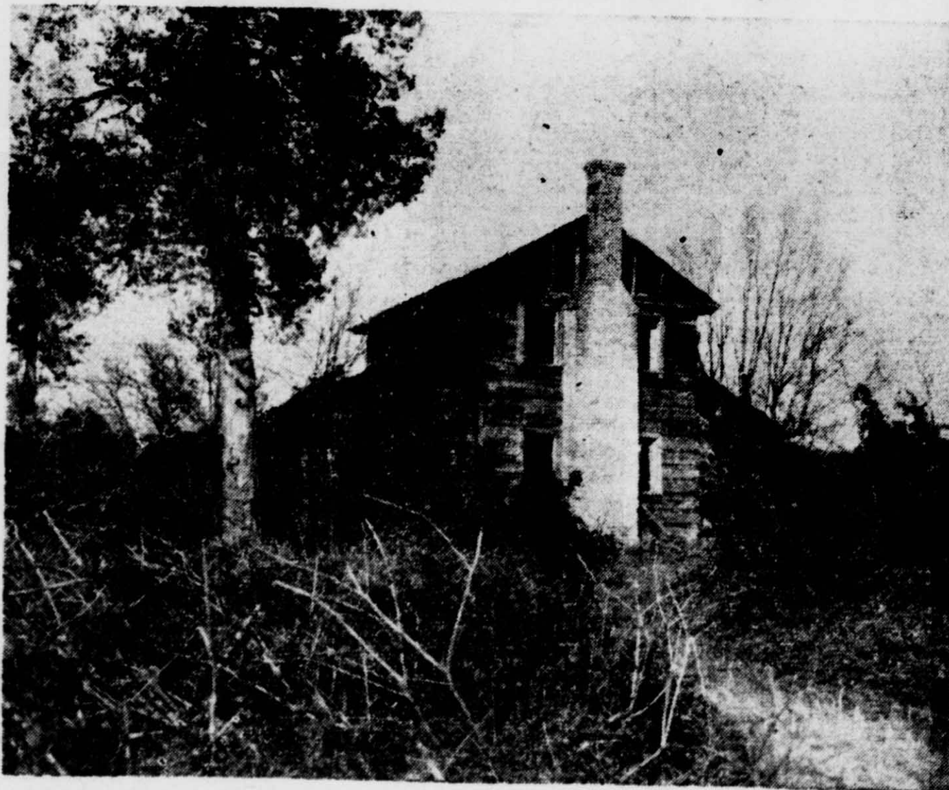
Sound timbers are still left in this old house in the King's Mountain State Park area, although no one has lived in it for years. The chimney seen in the foreground is strong and usable but the one opposite has crumbled and lies partly within the rooms of the home. (Herald Staff Photo).
