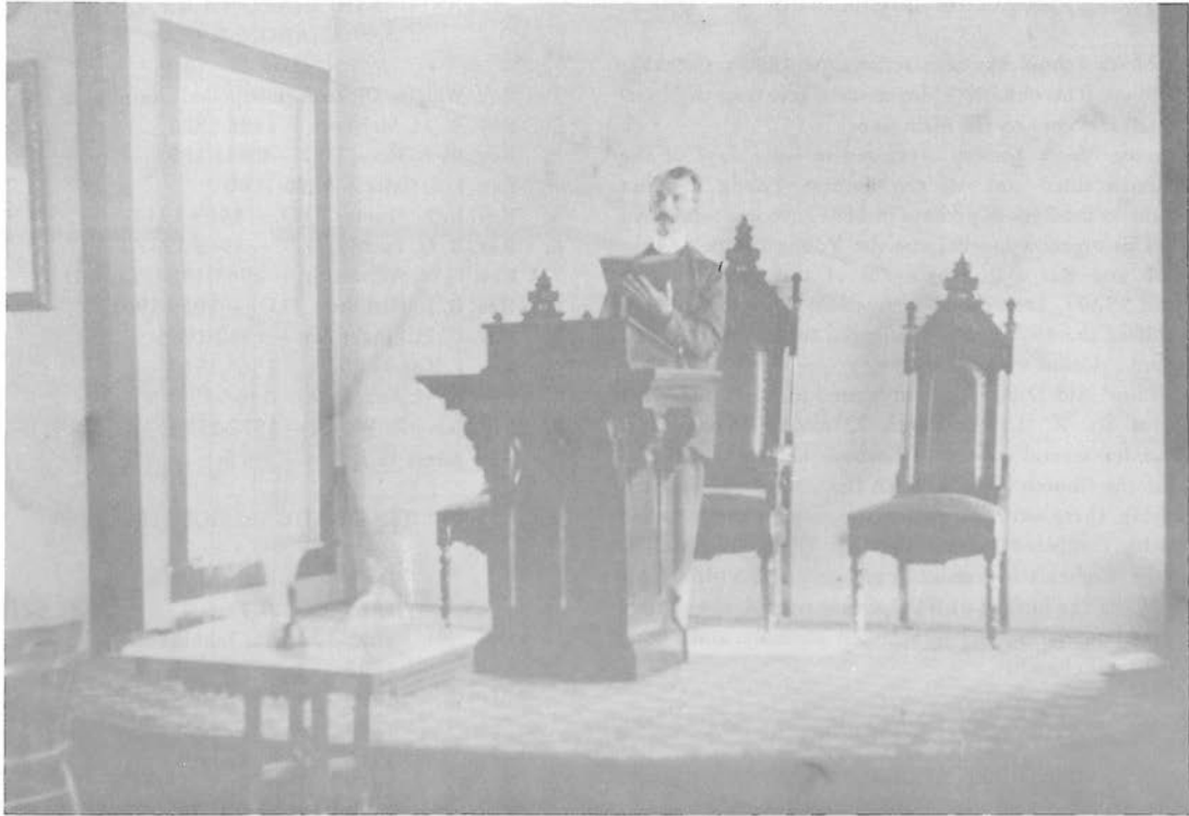
Rev. J. S. Grier in pulpit. Interior of Old Church
