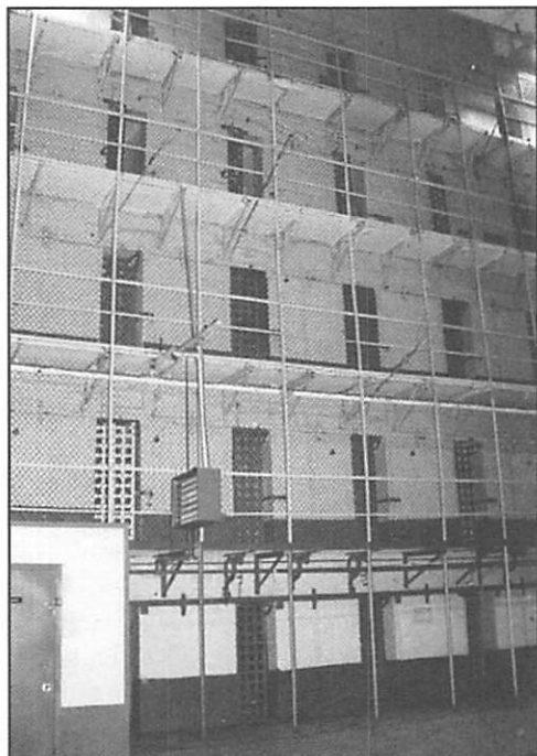
Late-twentieth-century photograph of the interior of the South Carolina Penitentiary's North Wing Cell Block. Completed in 1886, the five-story, granite building was designed to house 250 convicts. Aside from the grating on the catwalks opposite the cell doors and the small room in the foreground, the photograph reveals very few alterations to the original construction. Courtesy of the South Carolina Department of Archives and History, Columbia.
