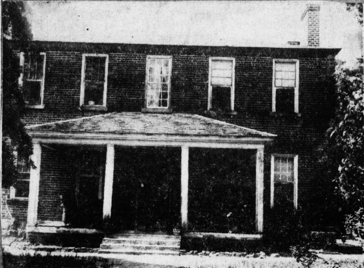
PROFESSOR'S HOME —This old building formed a part of Furman University when it was located at Winnsboro. It was used as a "professor's home" during that period. Across the highway to the south, still stands one of the old school buildings. It was originally a three-story brick structure, but the third story was damaged in the Charleston earthquake of 1886 and the top story was removed. (Observer Staff Photo by Hancock).
