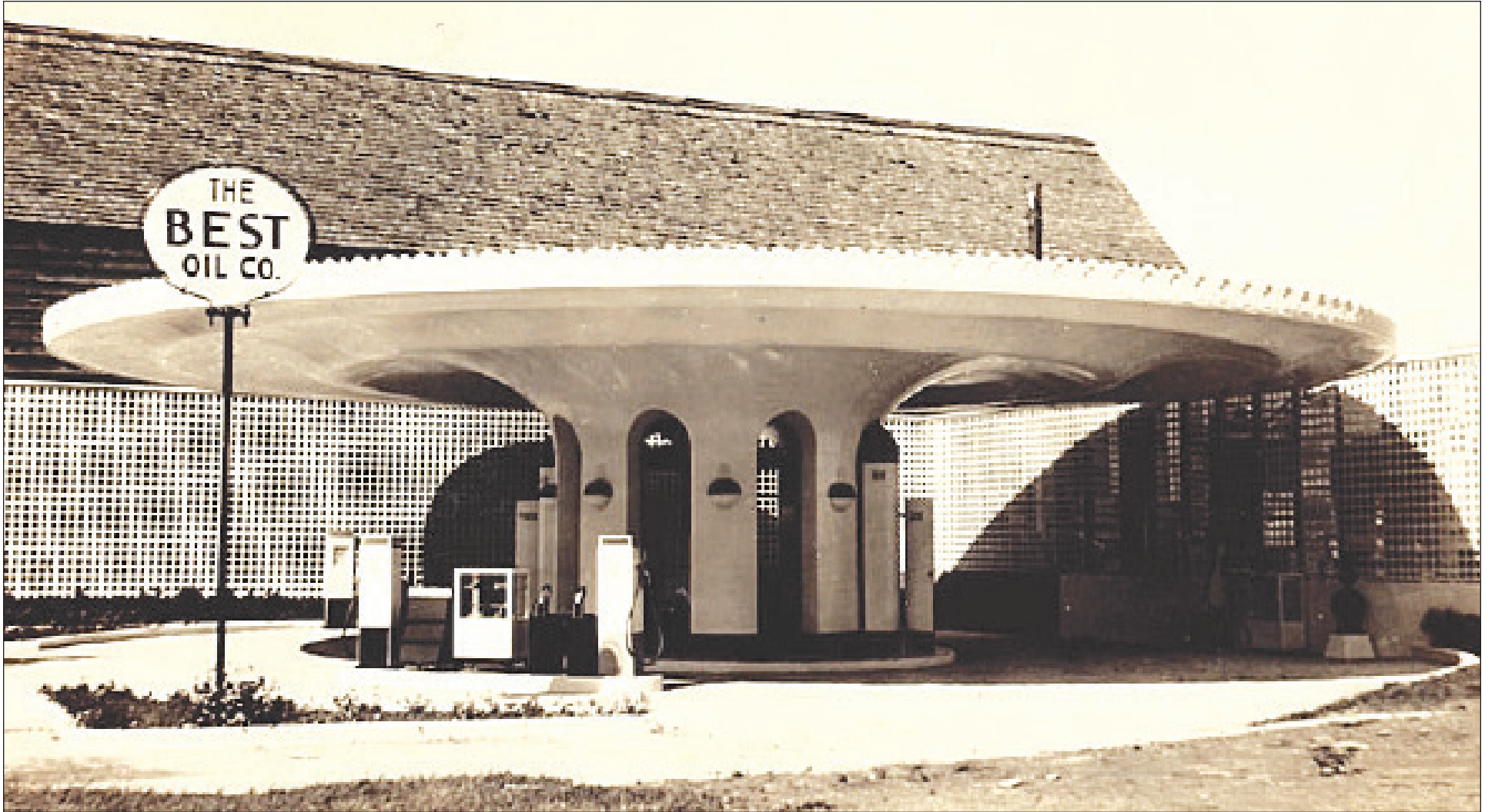
As described in a 1938 issue of The State newspaper, 'This new type station consists of a center column, containing rest rooms, office, meters and of a circular canopy of reinforced concrete extending as much as 40 feet outward from the column, unsupported by additional props, thus allowing motorists to drive in and out with ease. Gasoline nozzles are pulled down from overhead. The thing resembles a huge, flat umbrella and it represents what seems to be an important triumph in the art of concrete work.'
