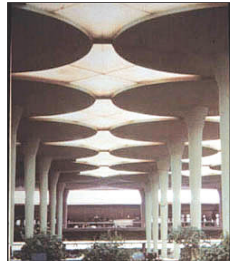
Frank Lloyd Wright's famous dendri-form columns in the S.C. Johnson Wax building in Racine, Wisc., are strikingly similar to the design of a service station built earlier in Winnsboro by architect James Workman.
