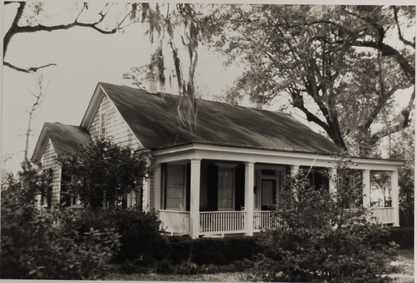
Photo # Photo Index # View of N, S, E, W 1 D6, F15 Facade & Left E
