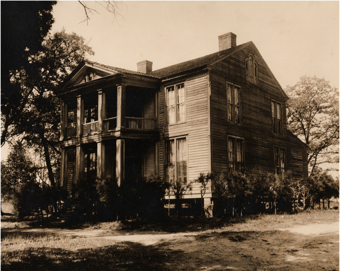
Mount Holly , cir. 1850. Hand hewn and pegged timbers, Rowells section, Eastern Chester Co.
