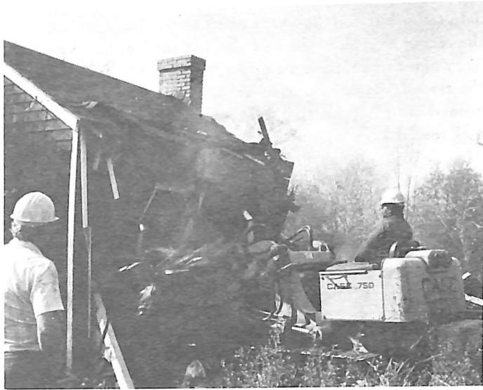
CREW "PUSHIN' DOWN" old abandoned house.
