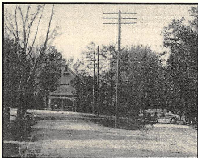
Bradley Home on Center Street
