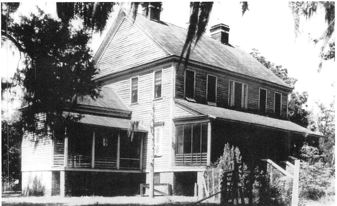
The Springfield mansion was constructed of black cypress. The house had six rooms on the first floor and a broad piazza stretched across the front.
